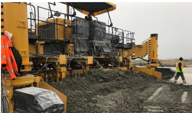
Picture 1: Concrete with MCE™ can be placed using traditional methods, including slipform paving.
